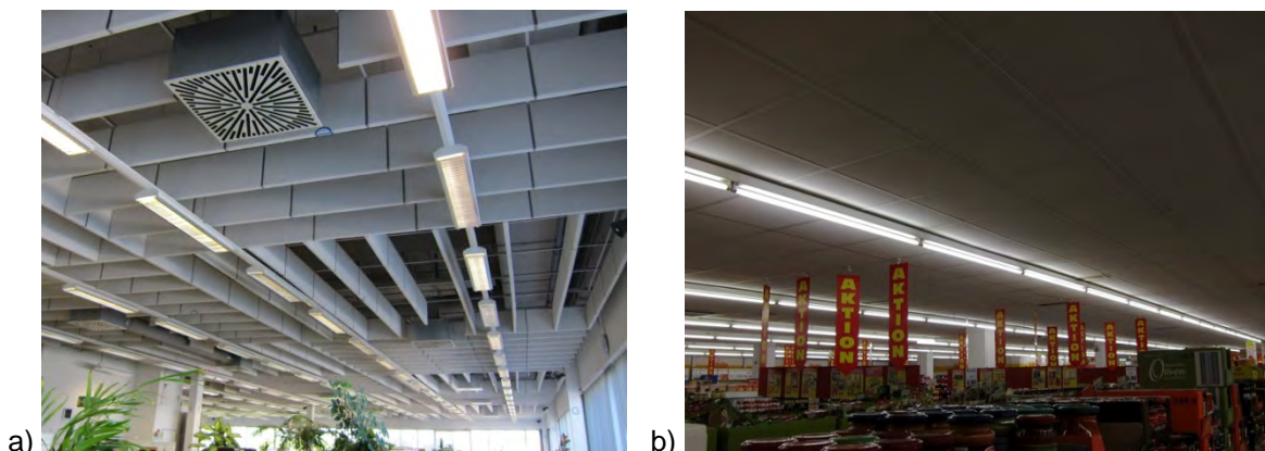
Figure 1: Lamp installations in open office space (a) and supermarkets (b).
