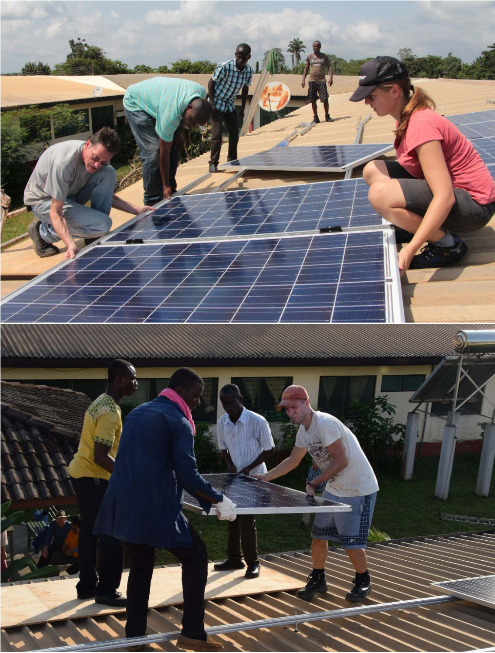
Installing a hybrid system in Ghana
